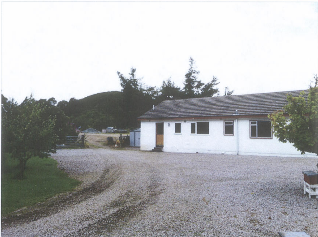
Image 04: Access to working farmyard from vehicle parking and turning area
