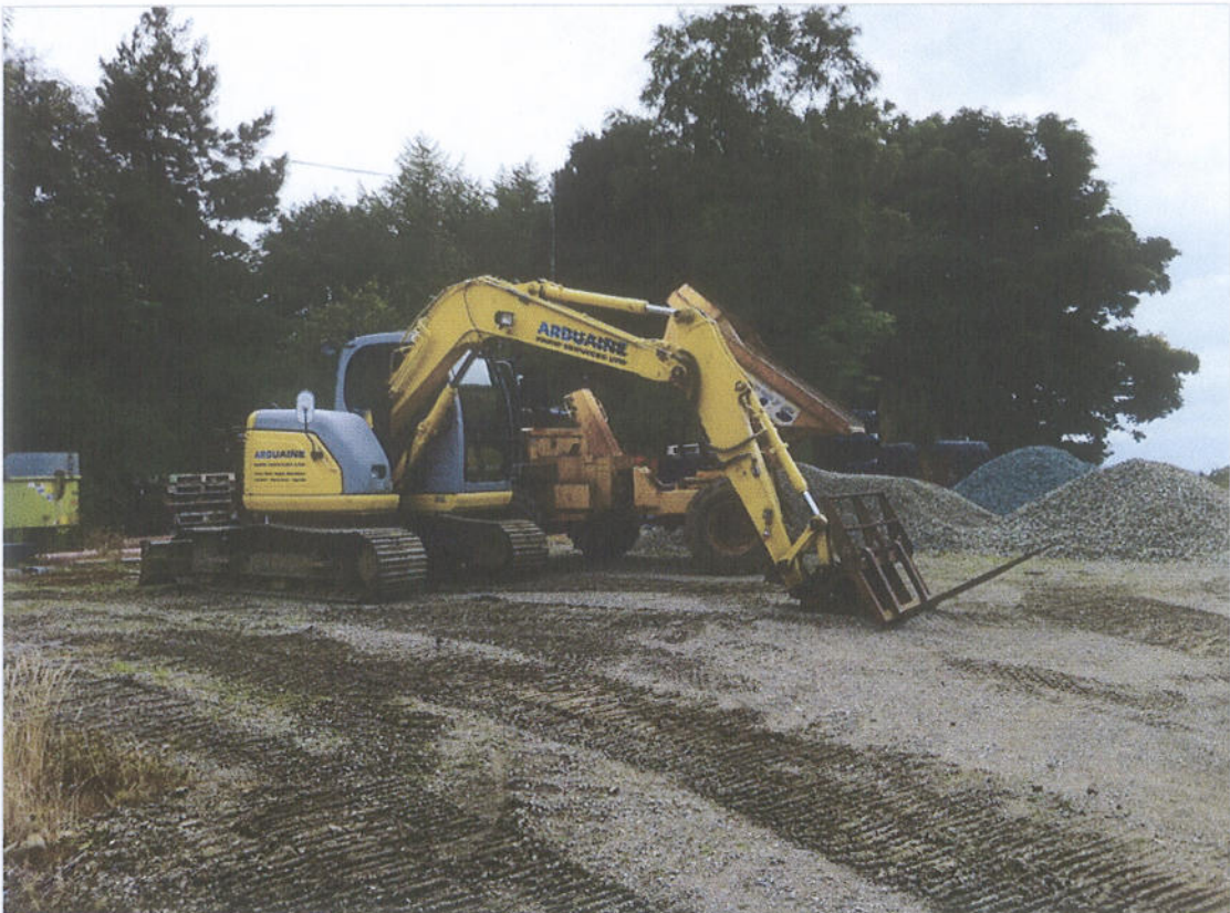
Image 08: Plant, equipment and materials storage area east
