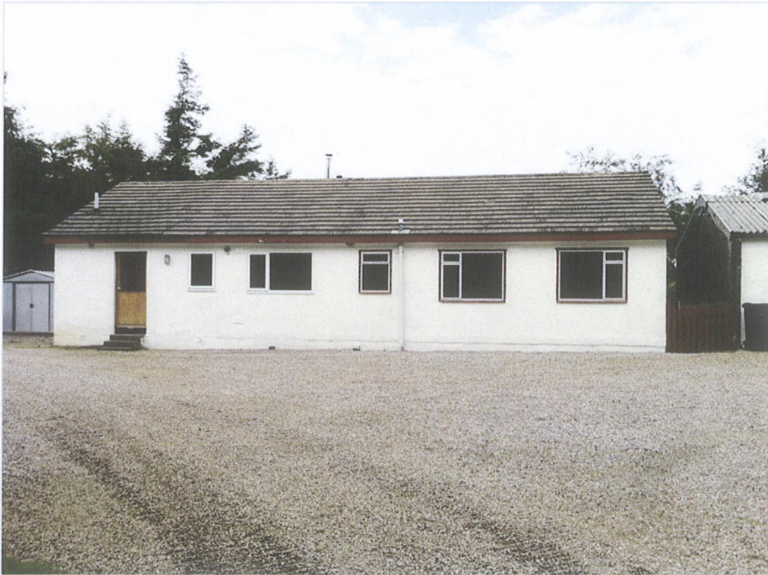
Image 03: Arduaine Farm House, Dorran pre-fabricated bungalow.
